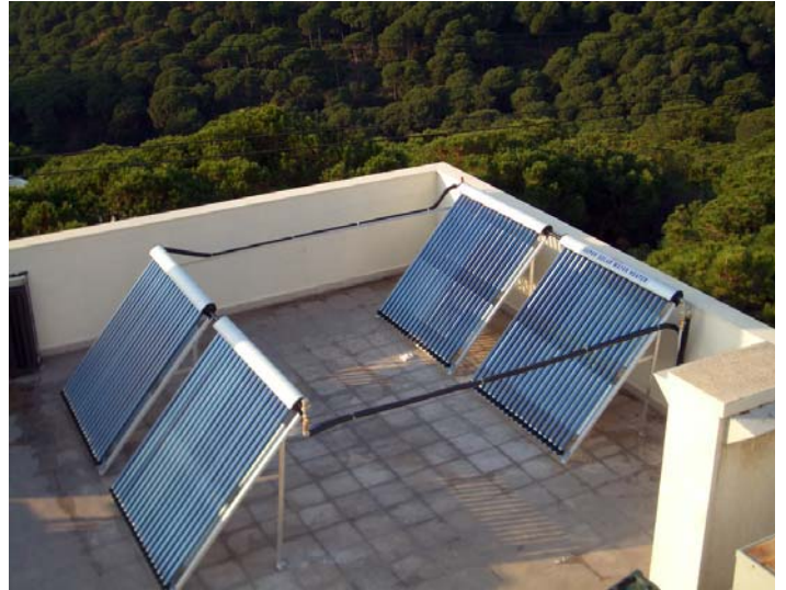
Evacuated tube Solar Hot Water Heating Systems
