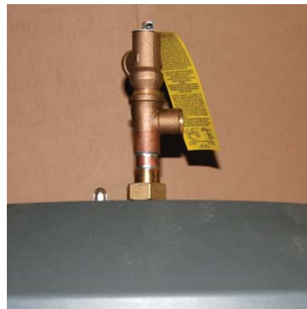
Complete assembly on SBB tank.
